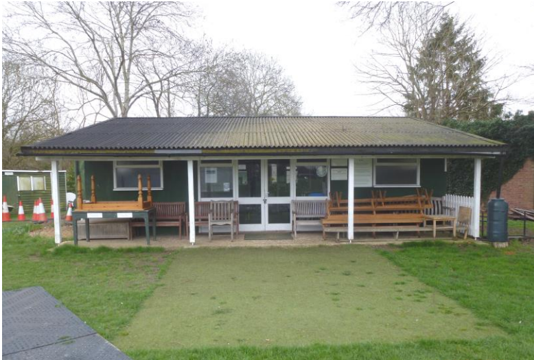
The pavilion to be demolished
