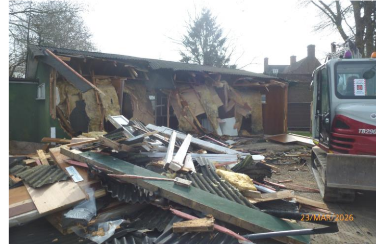
23.3.2026 Demolition work in progress
